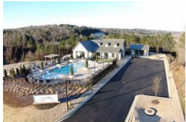
Capstone has finished work as general contractor on Easterwood.
